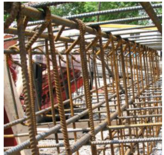
Rebar in place for reinforced concrete
